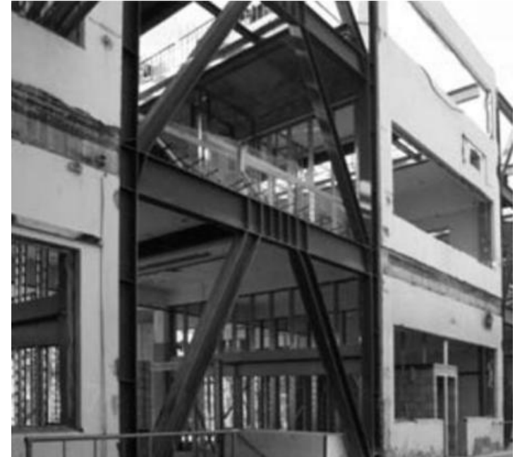
Eccentrically braced frames strengthen a reinforced concrete building
