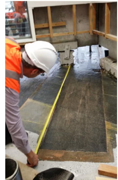
Slab strengthening with FRP (© Umut Akguzel)
