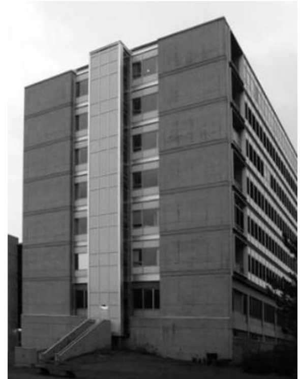
External retrofitted concrete shear walls (Charleson, 2008)
