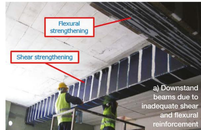
FRP for flexural and shear strengthening
