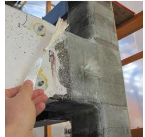
Installation of an FRP dowel through the bonded sheet into the beam.
