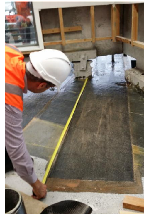
Site inspection of FRP slab strengthening (© Umut Akguzel)
