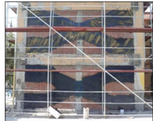
FRP-strengthened infill frame, Istanbul (Courtesy of OTS Eng. & Consultancy)
